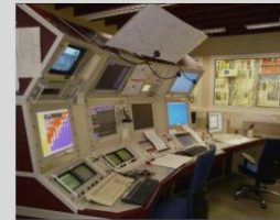
Operating console in Messhalle.
